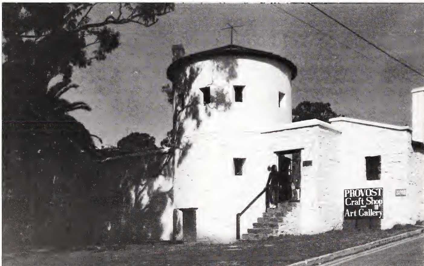
Fig 19. The Old Provost, built in 1838 for the incarceration of 20 Khoi soldiers, three of whom were executed for the murder of Ensign Crowe. The panopticon design for British prisons was the idea of the economist, Jeremy Bentham. The provost was restored in 1937.
